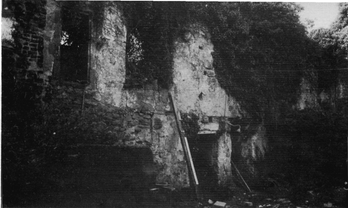
PLATE 2: The structure at the rear of Nos. 31-32 O'Connell Street, Clonmel.
